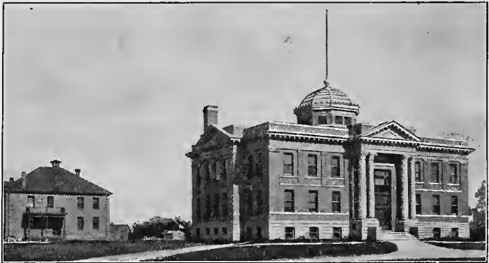
Courthouse, McHenry County
